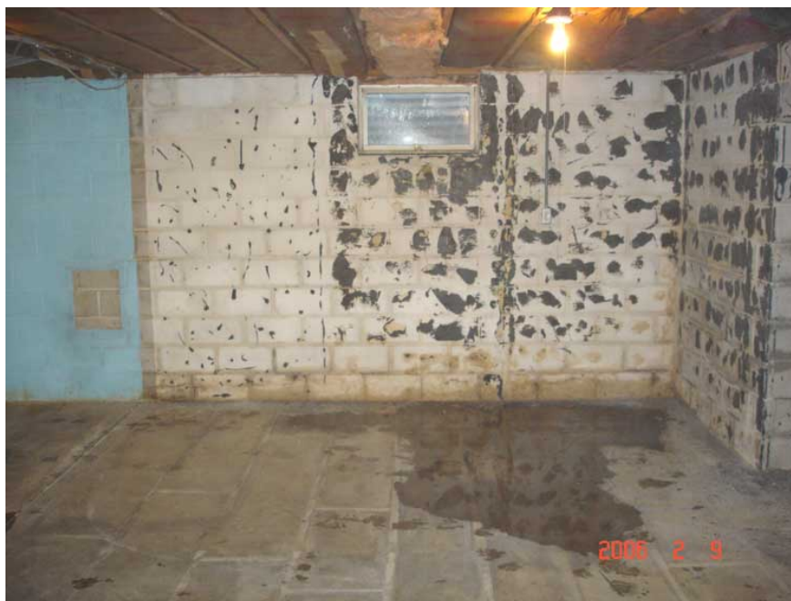
Mold and Mildew on the walls of a home
